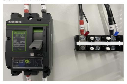
4. Turn on the input circuit breaker, fan circuit breaker, and output circuit breaker in sequence.
