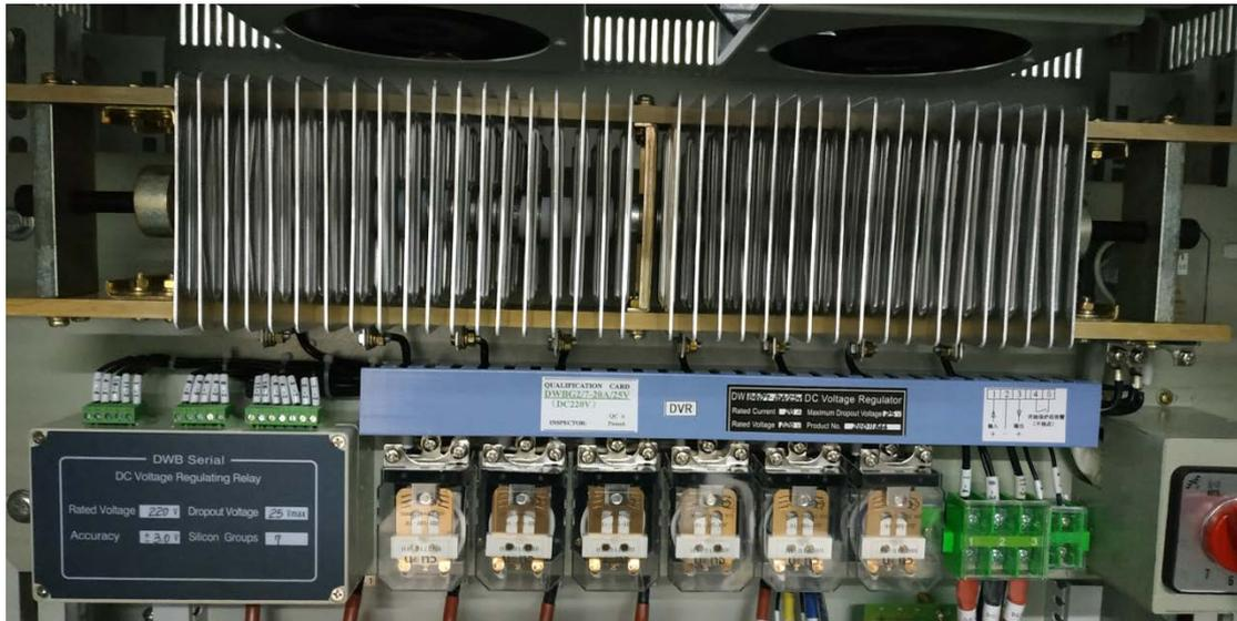
for dropping diode in picture, the model is DWBG2/7-20A/25V(DC220V):
